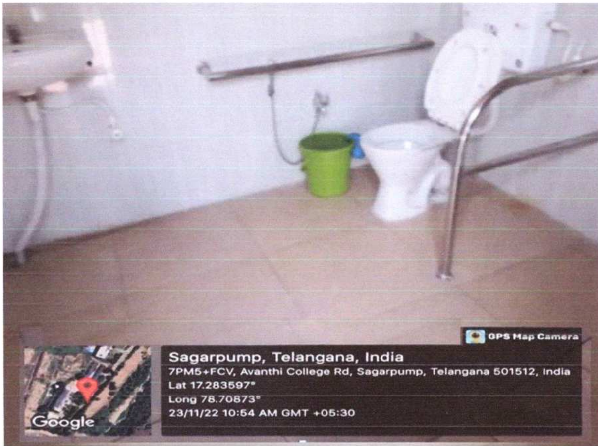
DIFFERENTLY ABLED FRIENDLY RESTROOM
