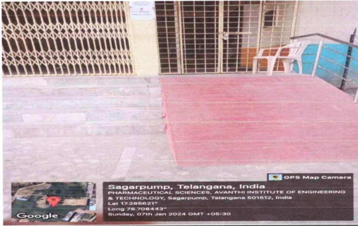
Ramps for Disabled Friendly Environment
